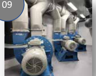
Frequency (VLT) controlled blowers
