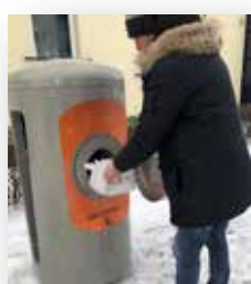
Outdoor Inlet (ODI) with Bluetooth Or RFID User ID option
