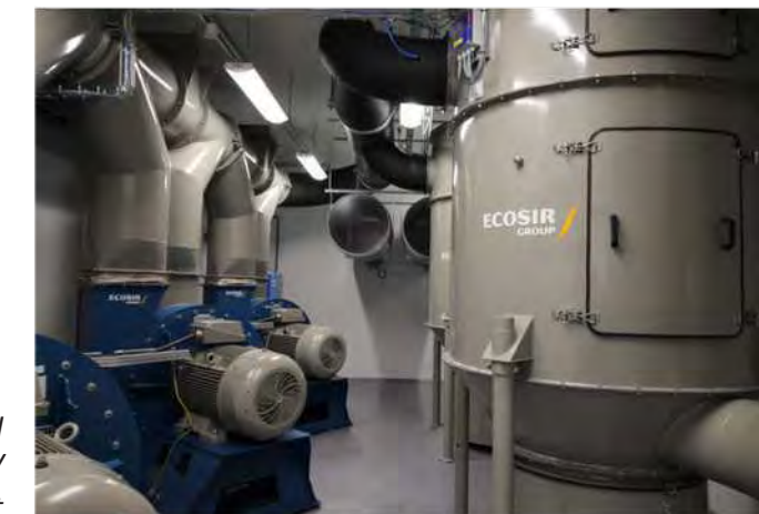
Compact and fully sealed filter/ blower room concept
