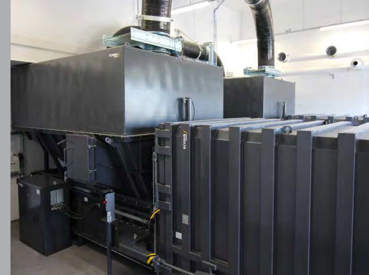
Powered motorised horizontal waste/air separation system – only 3.9 metres high!
