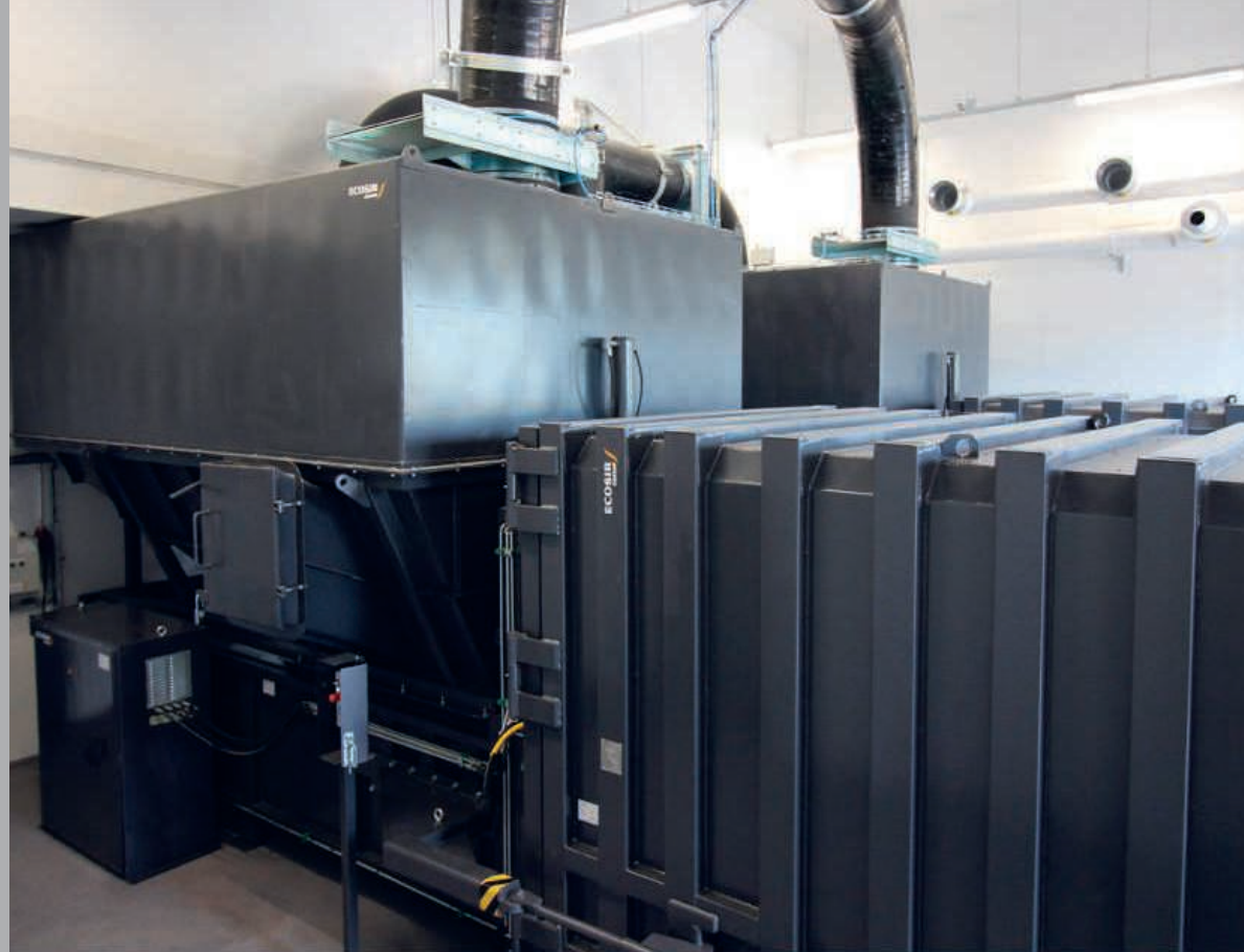
Powered motorised horizontal waste/air separation system – only 3.9 metres high!
