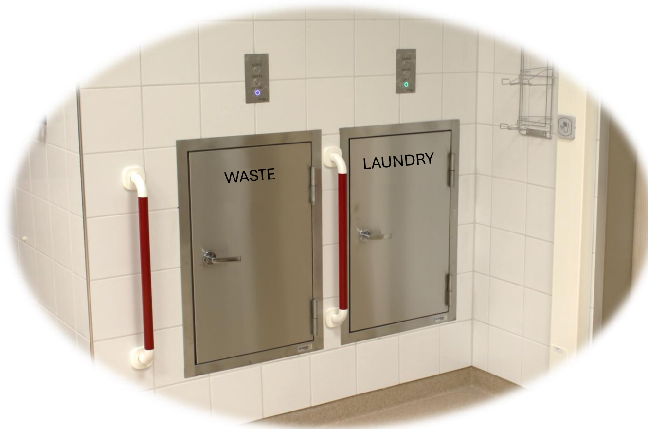
Picture: Drop&Go inlets with user control panels
