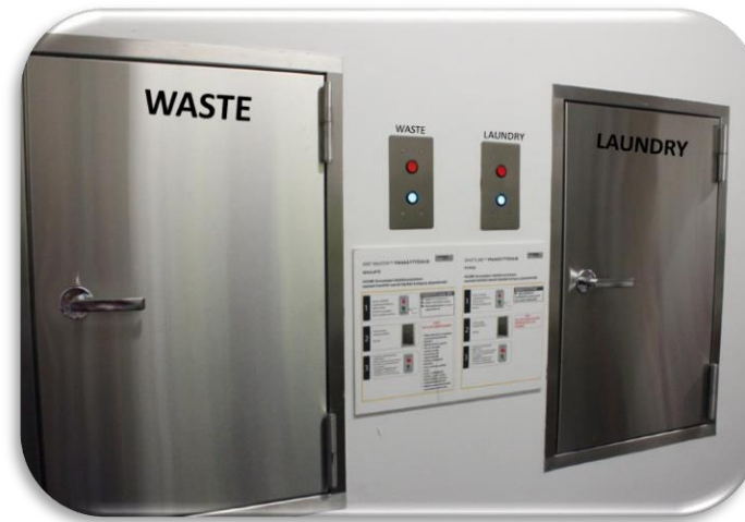
Picture: Drop&Go inlets with user control panels (LED button and info panel)
